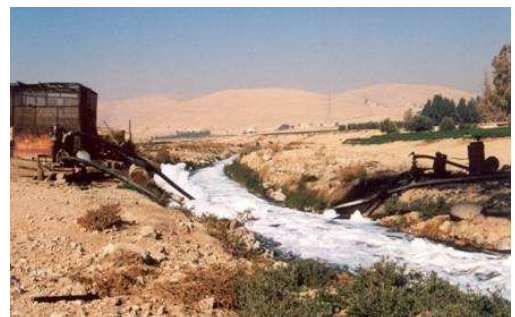
Use of sewage for irrigation (Amman, Jordan)
